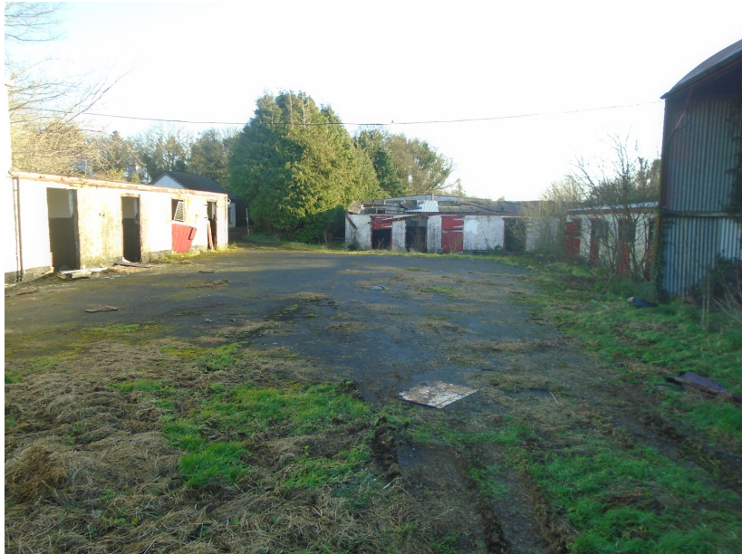
Plate 1 Outbuildings, looking E
